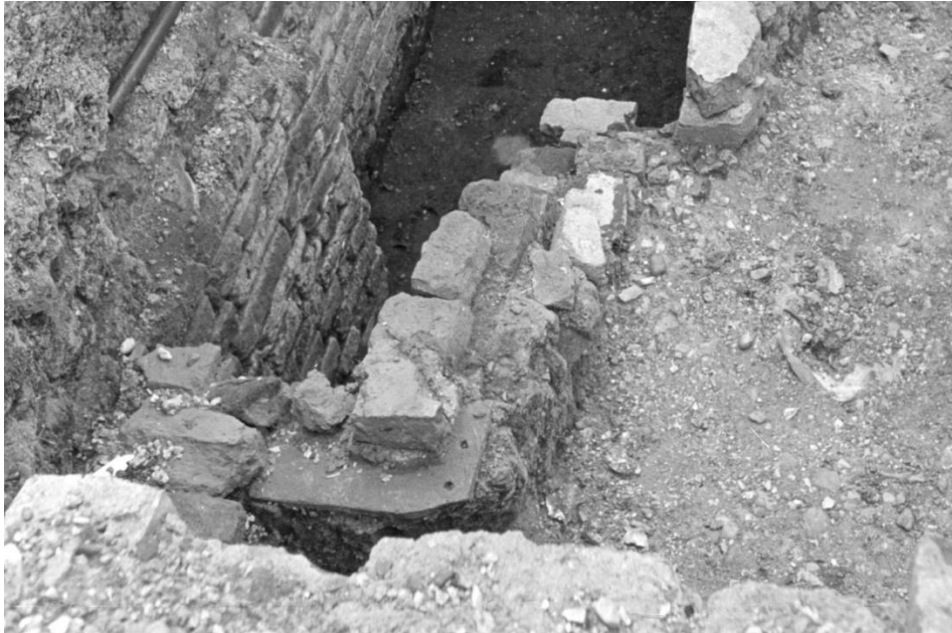
Pl. 11: PG77 Area I, Structure [1] Looking South Showing the Brickwork Above the Peg Tile at the North End Lost by the Time the Structure was Professionally Recorded (photo ?S. Somers/EAS Archives)
