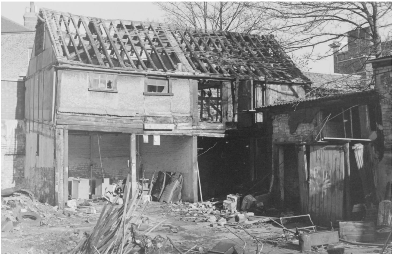
Pl. 20: Laing's Yard Barn Looking North During Demolition (photo G. Williams)
