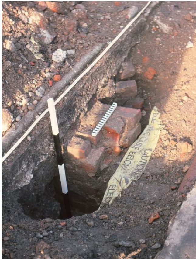
Pl. 17: Wall Exposure at Fig. 2 No. 4, Presumed to be Looking North (photo Ian K. Jones)
